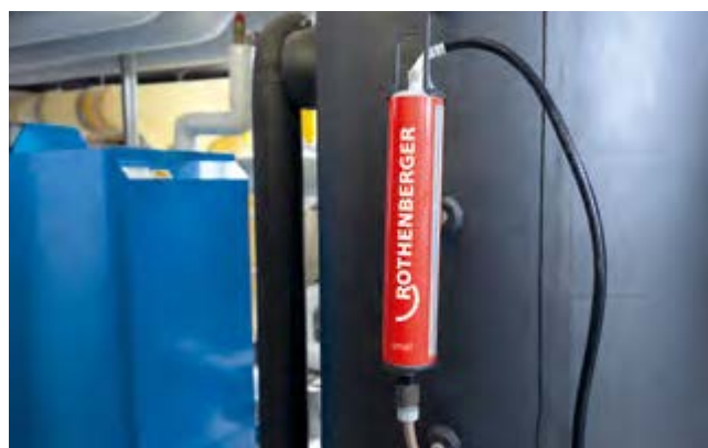
Set in size S with wall bracket and filling hose for the right station for demineralized water
