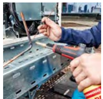
Brazing in refrigeration / air-conditioning technology
