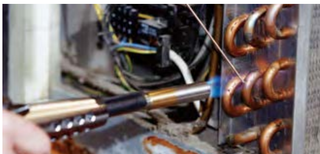
Brazing in refrigeration / air-conditioning technology
