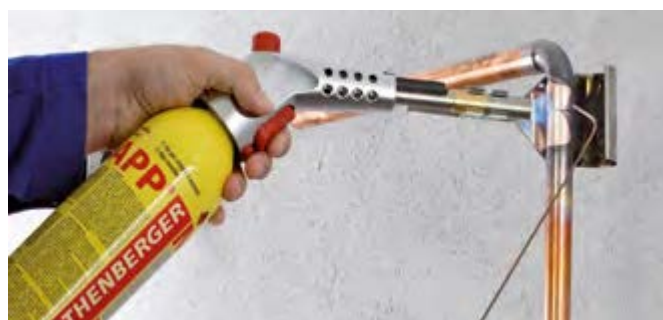
Brazing in gas installation
